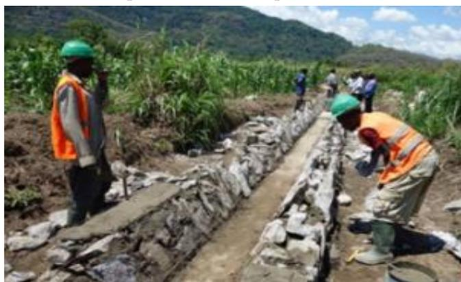
**Photo 3. Irrigation scheme construction underway in 2014.**
